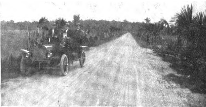
CAUSEWAY ON LA ROCHE AVENUE, A MODEL ROAD SURFACE.
